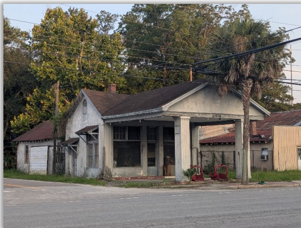
The abandoned 'Proctor Building'
