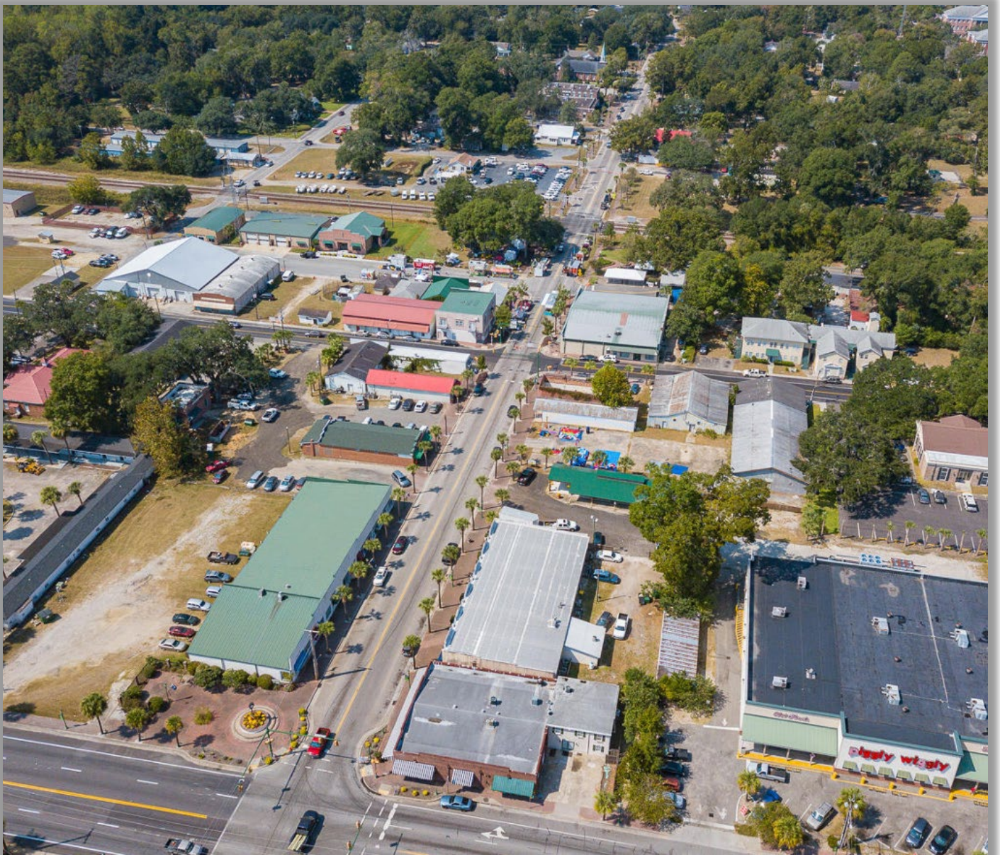
Aerial view of West Main Street
