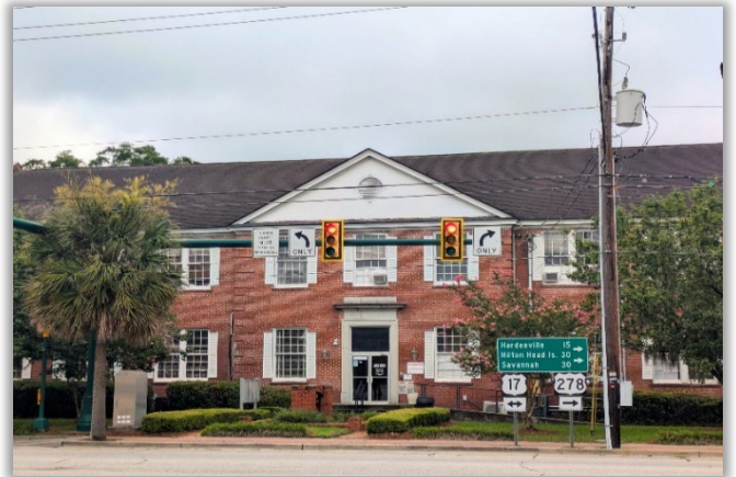
Jasper County School District building
