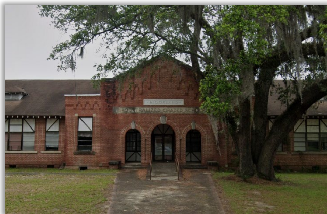
Ridgeland Centralized Graded School c.1928
