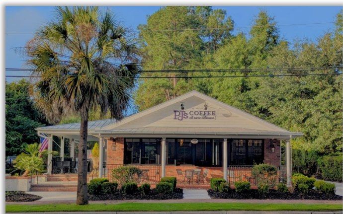
This house, c. 1950, was remodeled for PJ's Coffee while retaining its architectural character.
