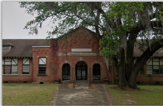
Ridgeland Centralized Graded School, c.1928
