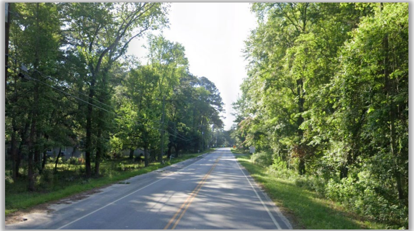
Grahamville Road is adjacent to the Exit 21 interchange, but this area has not been extensively developed.
