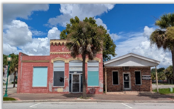
The old bank building on West Main Street, c.1925, is being targeted by the Ridgeland Development Group for rehabilitation.
