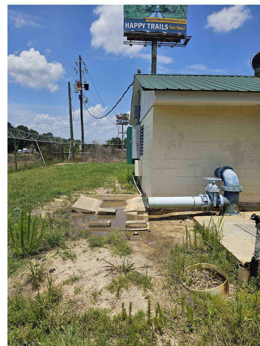
PHOTO 11: LOOKING NORTH TOWARD SPILLWAY CONCRETE AND DISCHARGE PIPE
