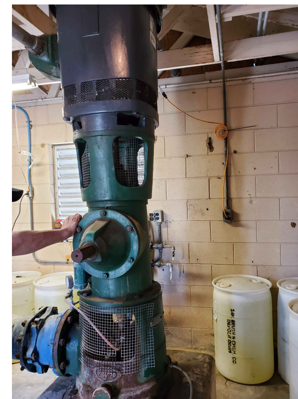
PHOTO 6: LOOKING WEST TOWARD WELL PUMP
