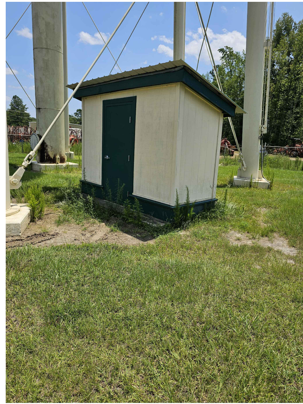
PHOTO 8: LOOKING EAST TOWARD ALTITUDE VALVE BUILDING
