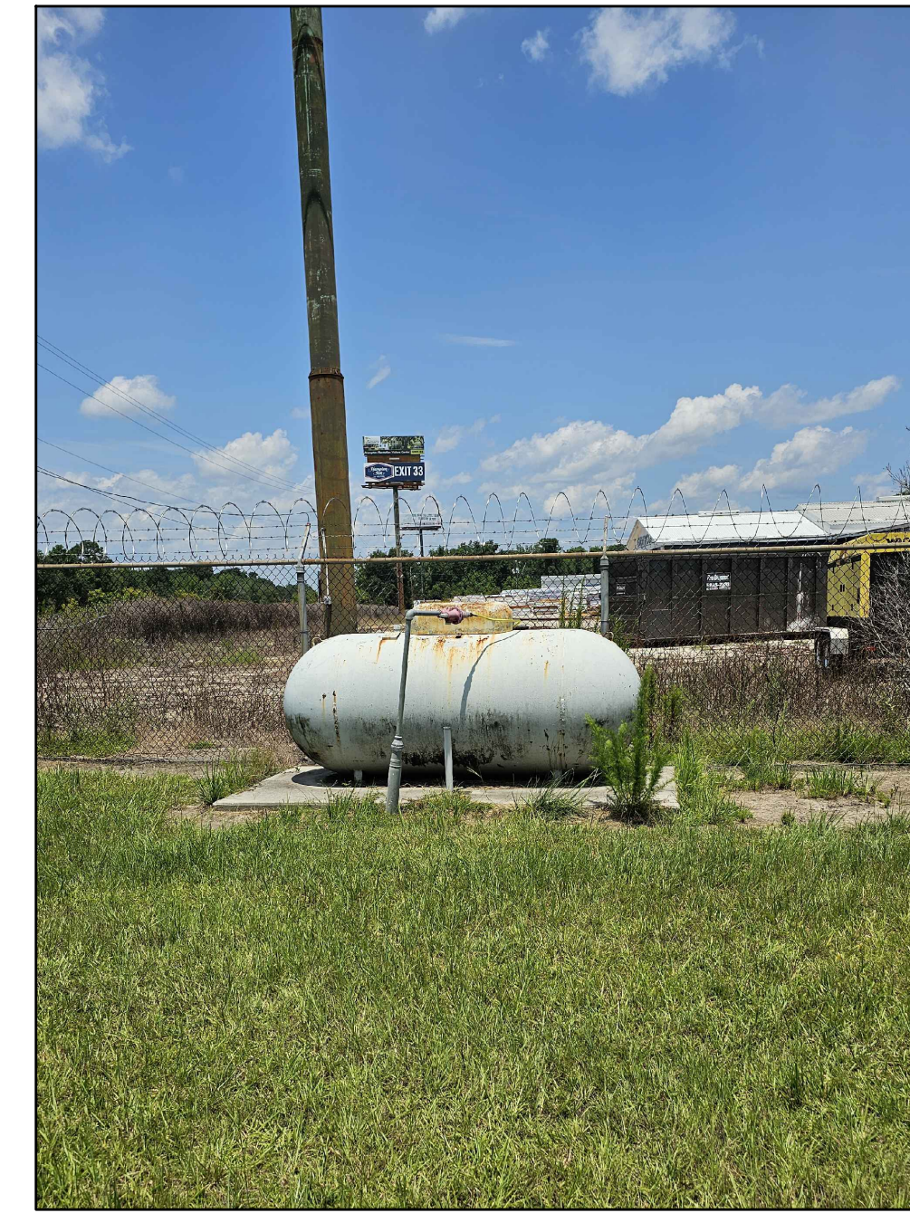
PHOTO 9: LOOKING NORTH TOWARD GAS TANK
