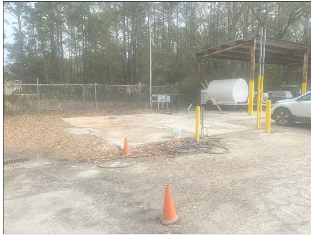
IMAGE-2 LOOKING NORTHEAST
