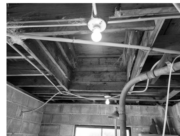
EXISTING ROOF ACCESS FRAMING
