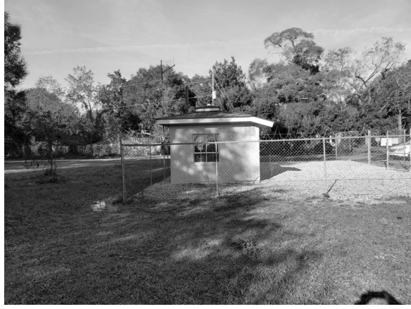
EXISTING LOOKING WEST
