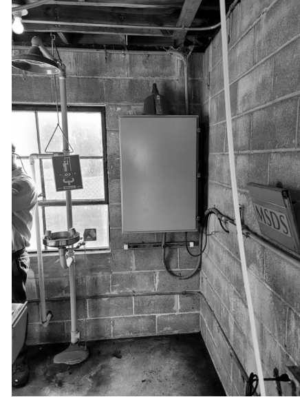
INTERIOR LOOKING EAST
