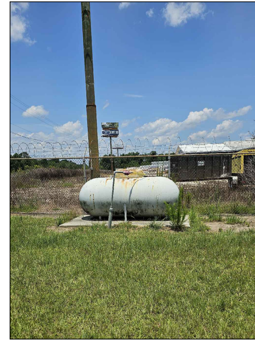
PHOTO 9: LOOKING NORTH TOWARD TOWARD GAS TANK
