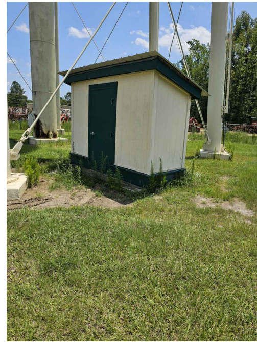
PHOTO 8: LOOKING EAST TOWARD ALTITUDE VALVE BUILDING
