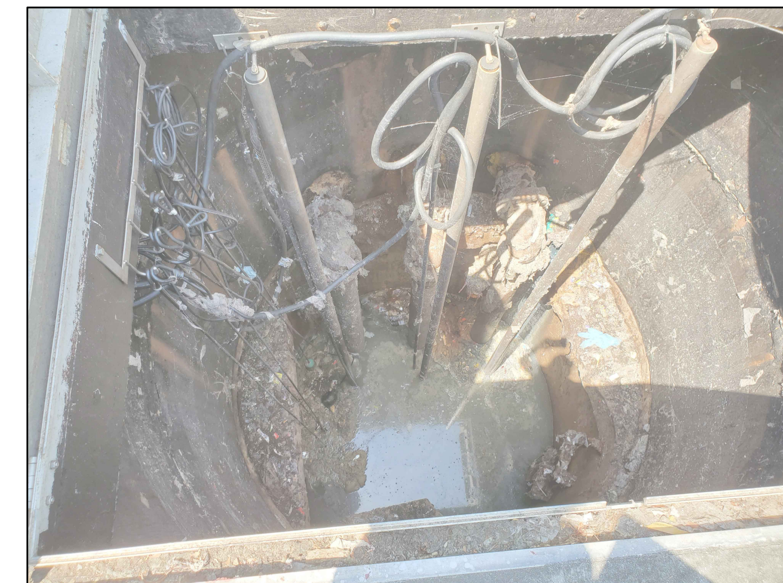
PHOTO-2 LOOKING DOWN IN WET WELL
