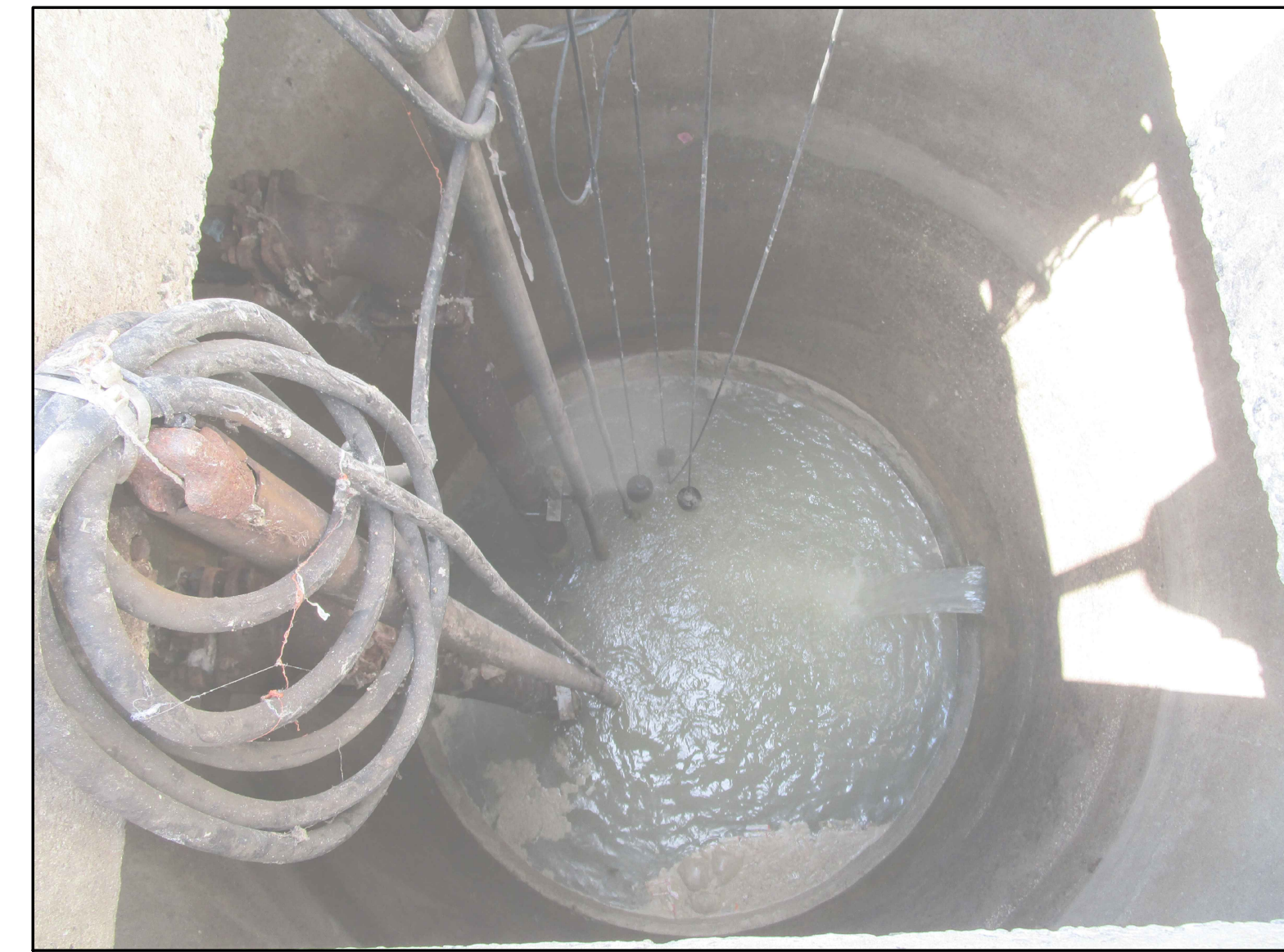
PHOTO-1 LOOKING INTO WET WELL
