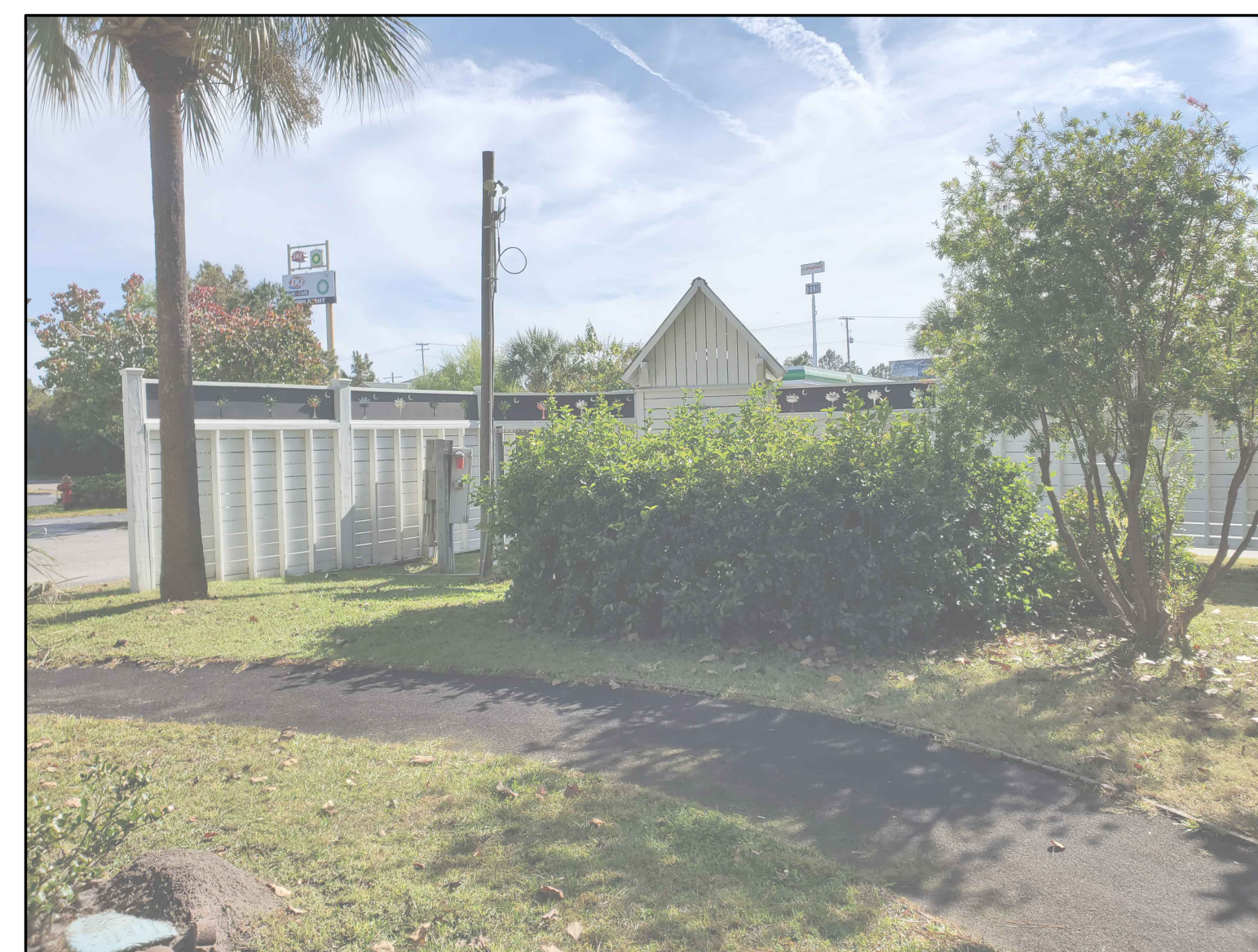
PHOTO-8 LOOKING SOUTH TOWARDS PS-4 FROM GARDEN/PARK
