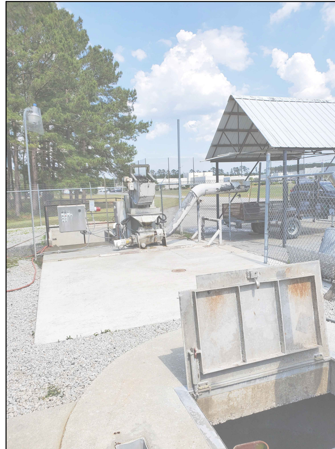
PHOTO-5 LOOKING EAST TOWARDS INFLUENT SCREENING FROM WET WELL
