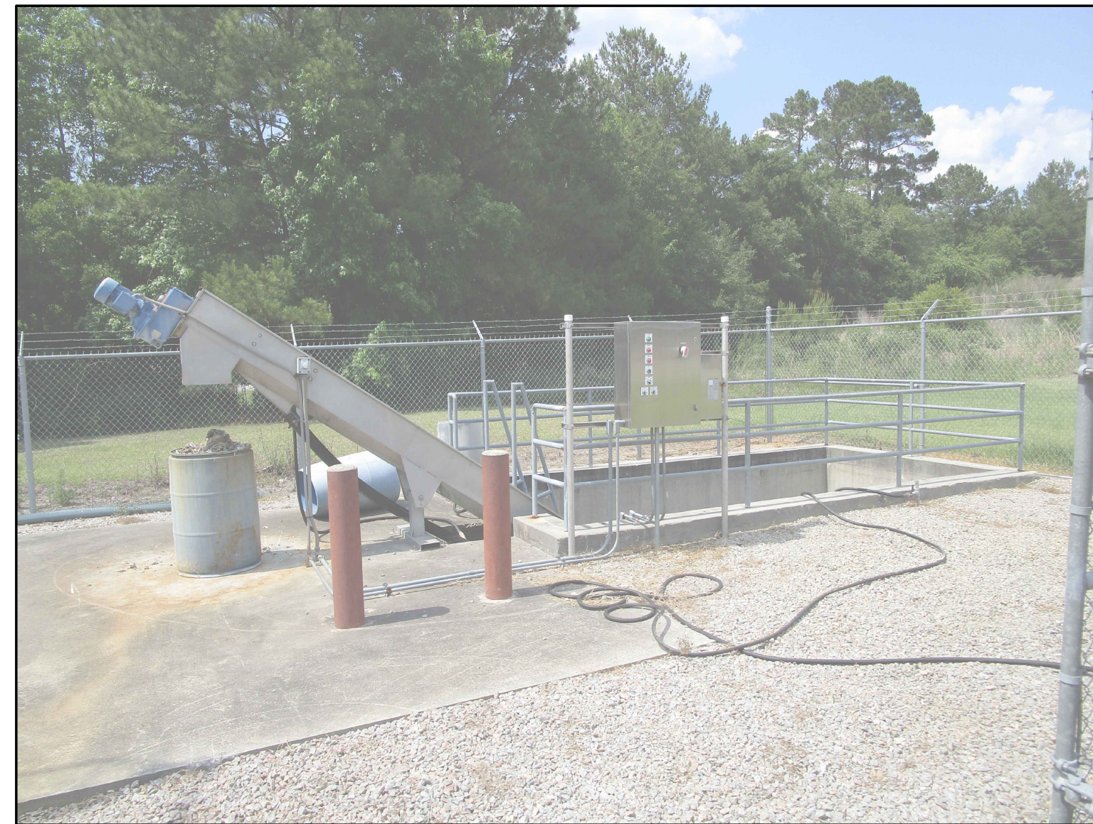
PHOTO-5 LOOKING NORTH AT SCREENING AREA OF SITE
