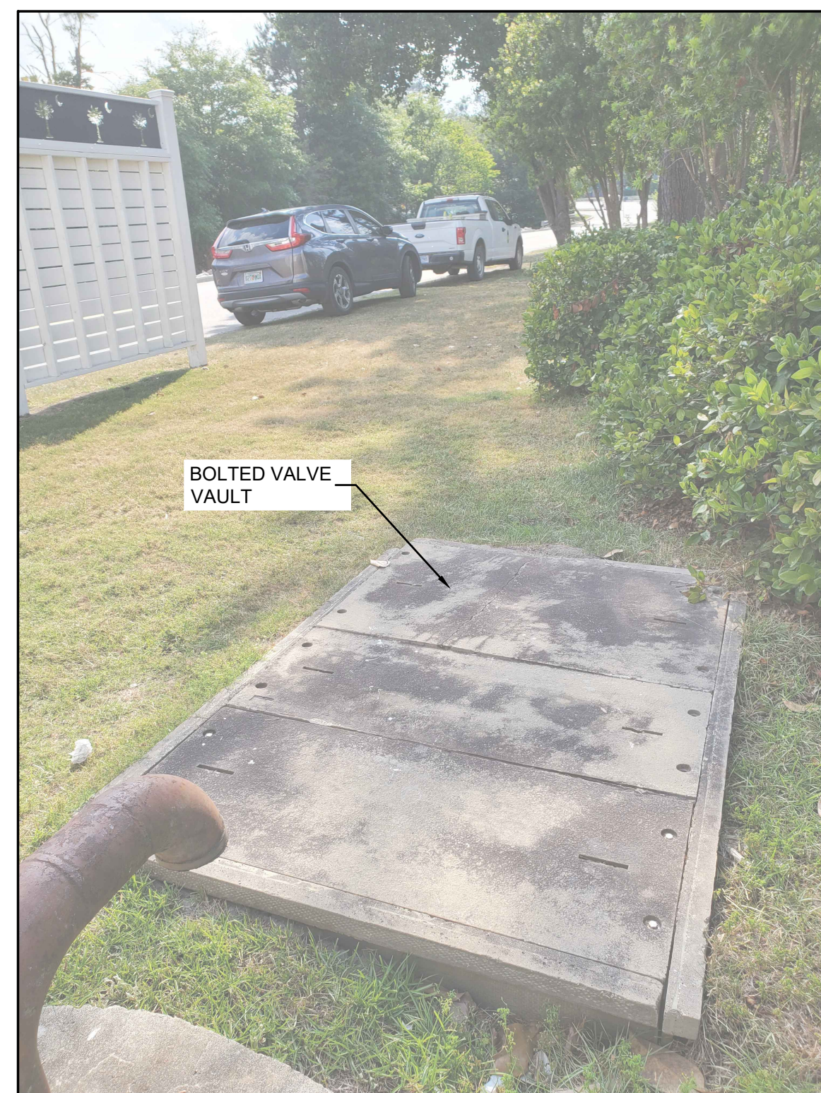
PHOTO-7 LOOKING WEST OVER VALVE VAULT
