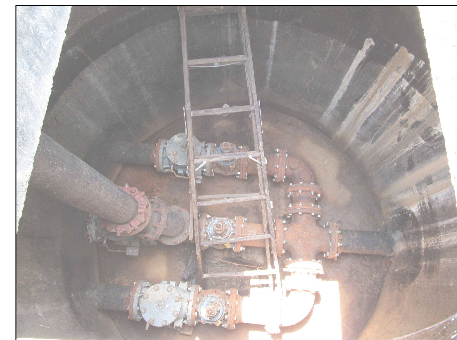
PHOTO-3 LOOKING DOWN IN VALVE VAULT
