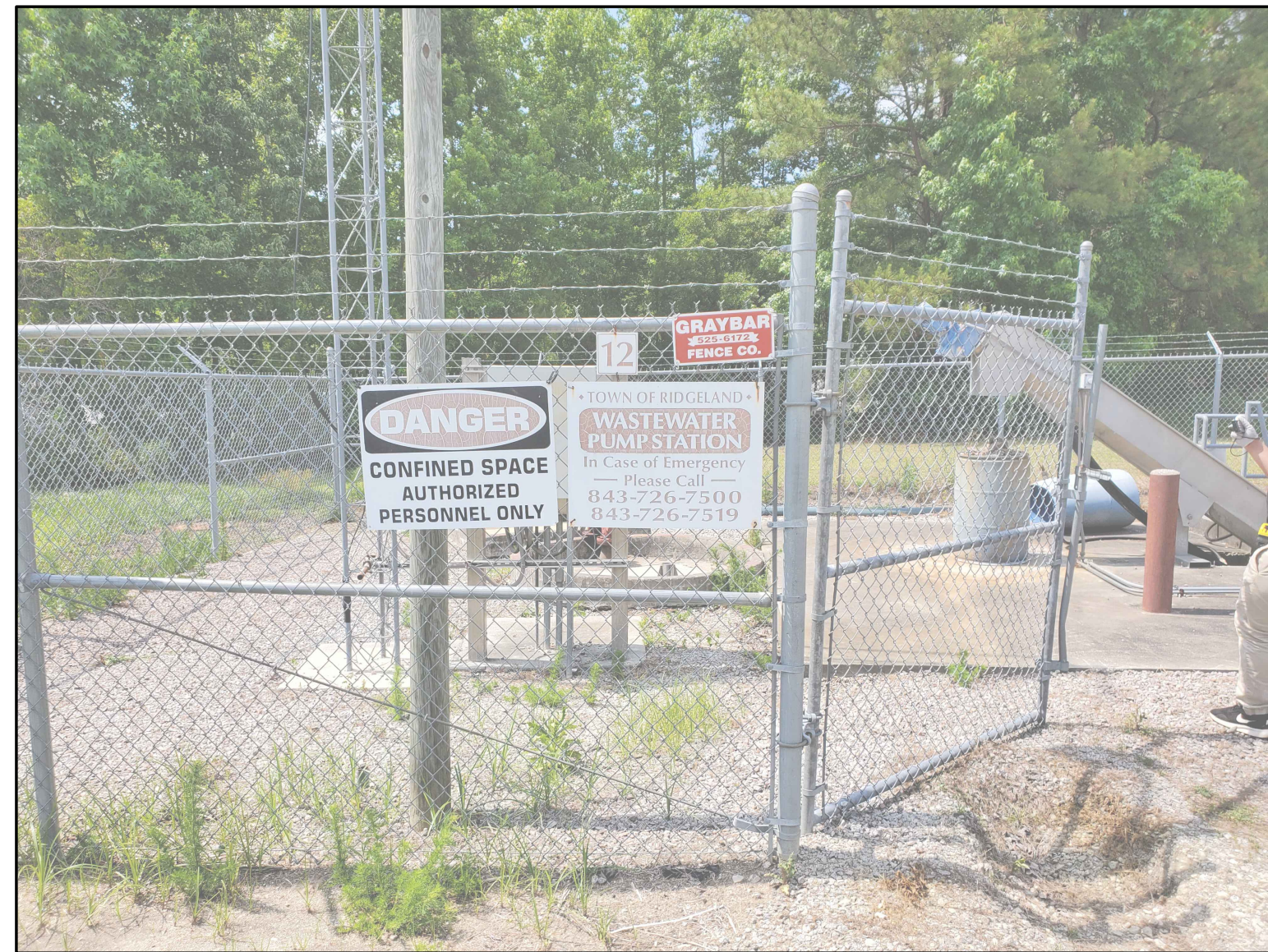
PHOTO-4 LOOKING NORTH AT PUMP STATION SITE
