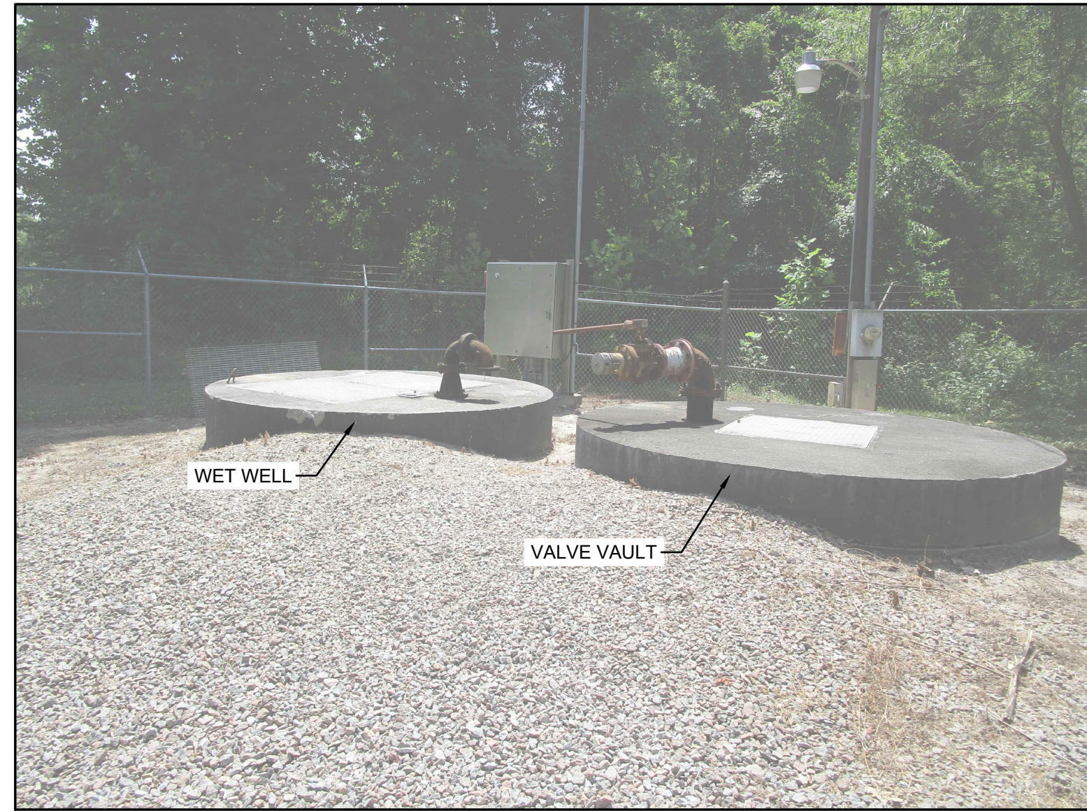
PHOTO-4 LOOKING SOUTHEAST AT WET WELL AND VALVE VAULT
