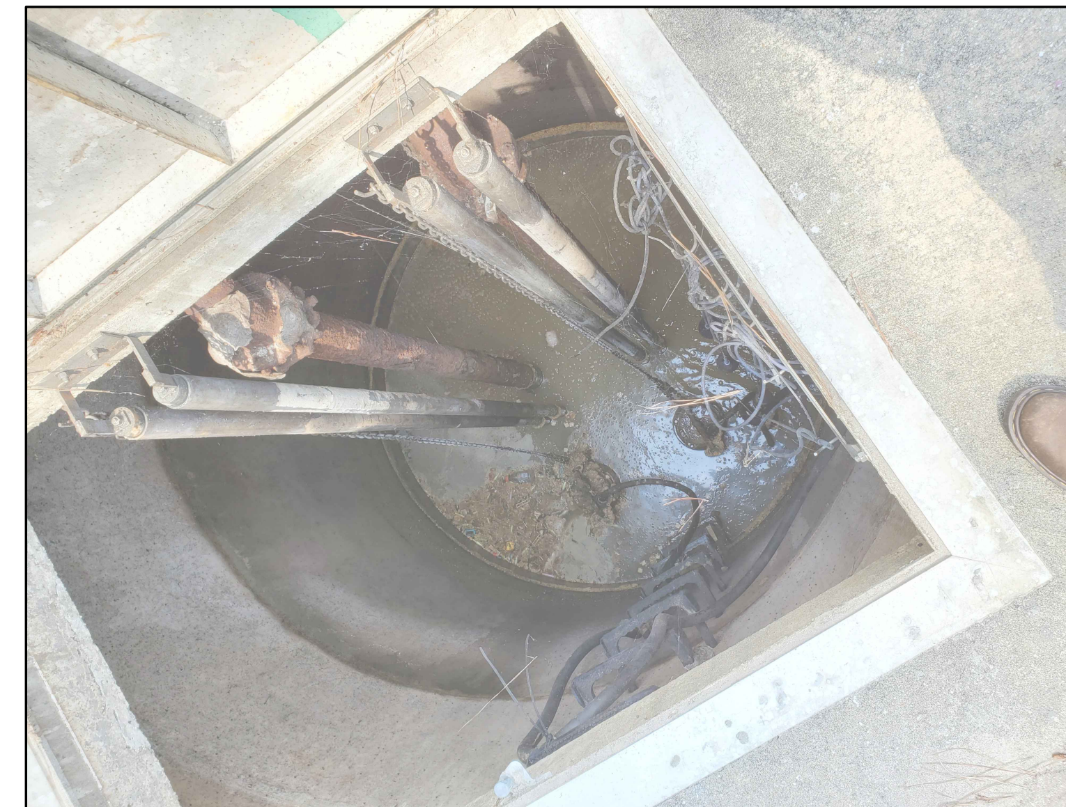
PHOTO-1 LOOKING INTO WET WELL
