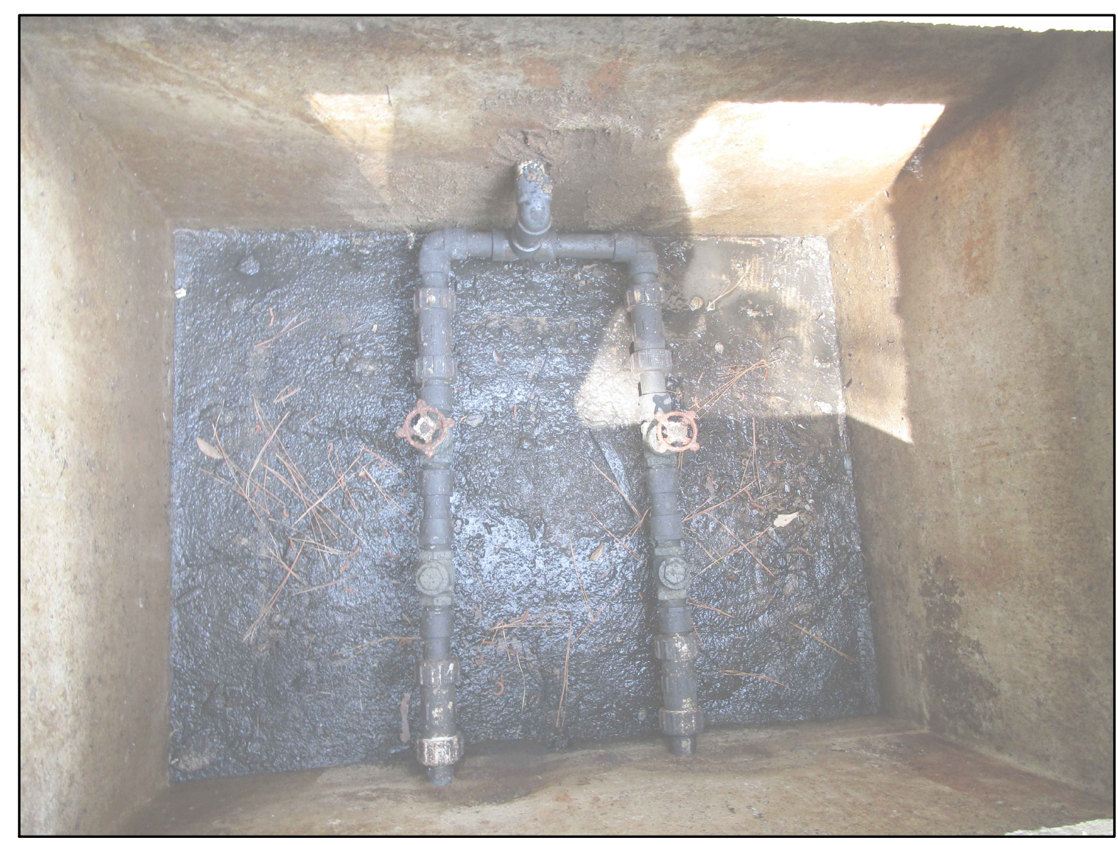
PHOTO-3 LOOKING INTO VALVE VAULT
