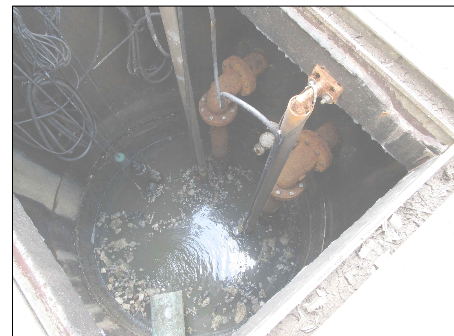
PHOTO-2 LOOKING INTO WET WELL
