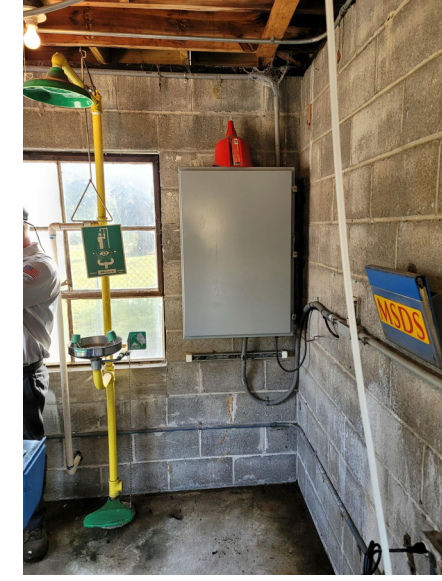
INTERIOR LOOKING EAST
