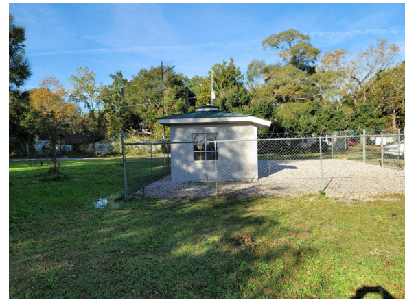
EXISTING LOOKING WEST
