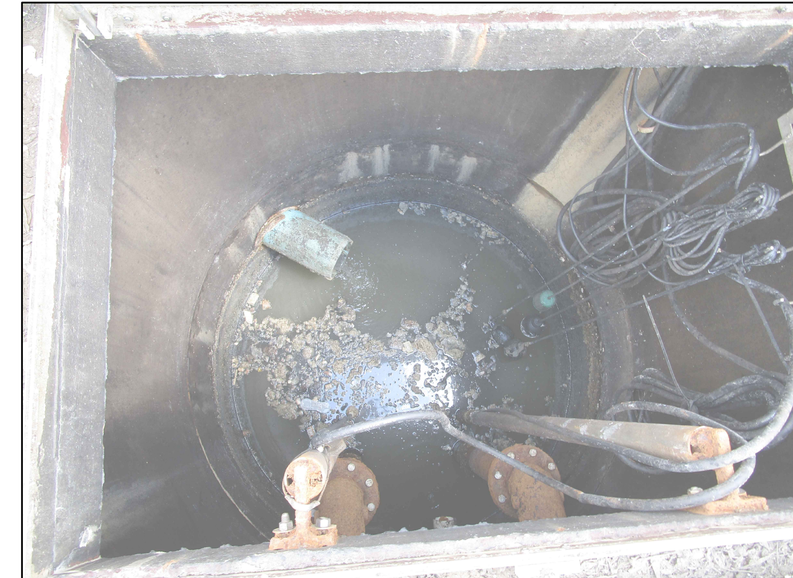
PHOTO-1 LOOKING INTO WET WELL
