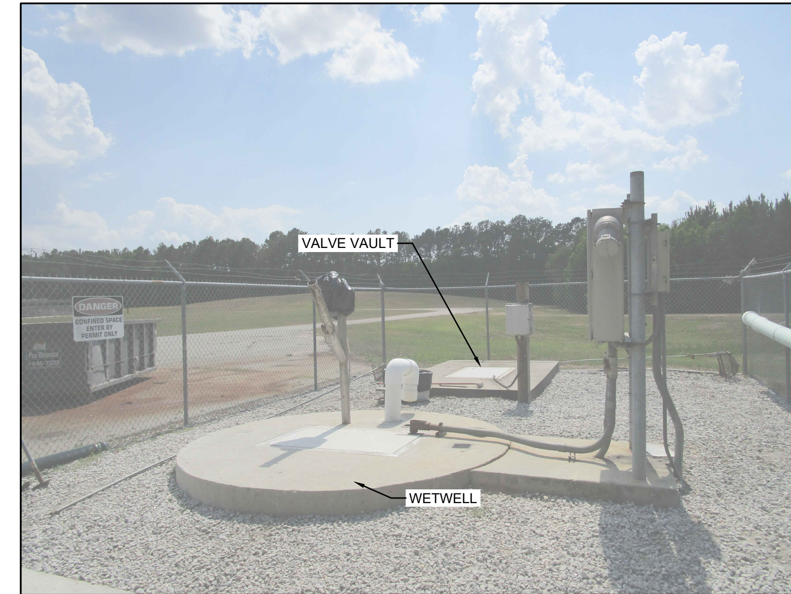
PHOTO-6 LOOKING WEST TOWARDS PUMP STATION
