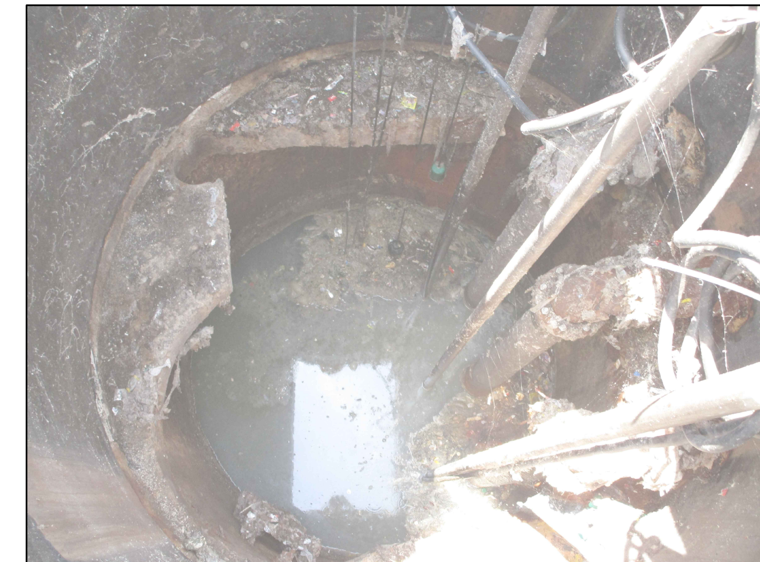
PHOTO-1 LOOKING DOWN IN WET WELL
