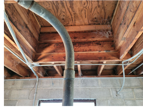
EXISTING ROOF ACCESS FRAMING
