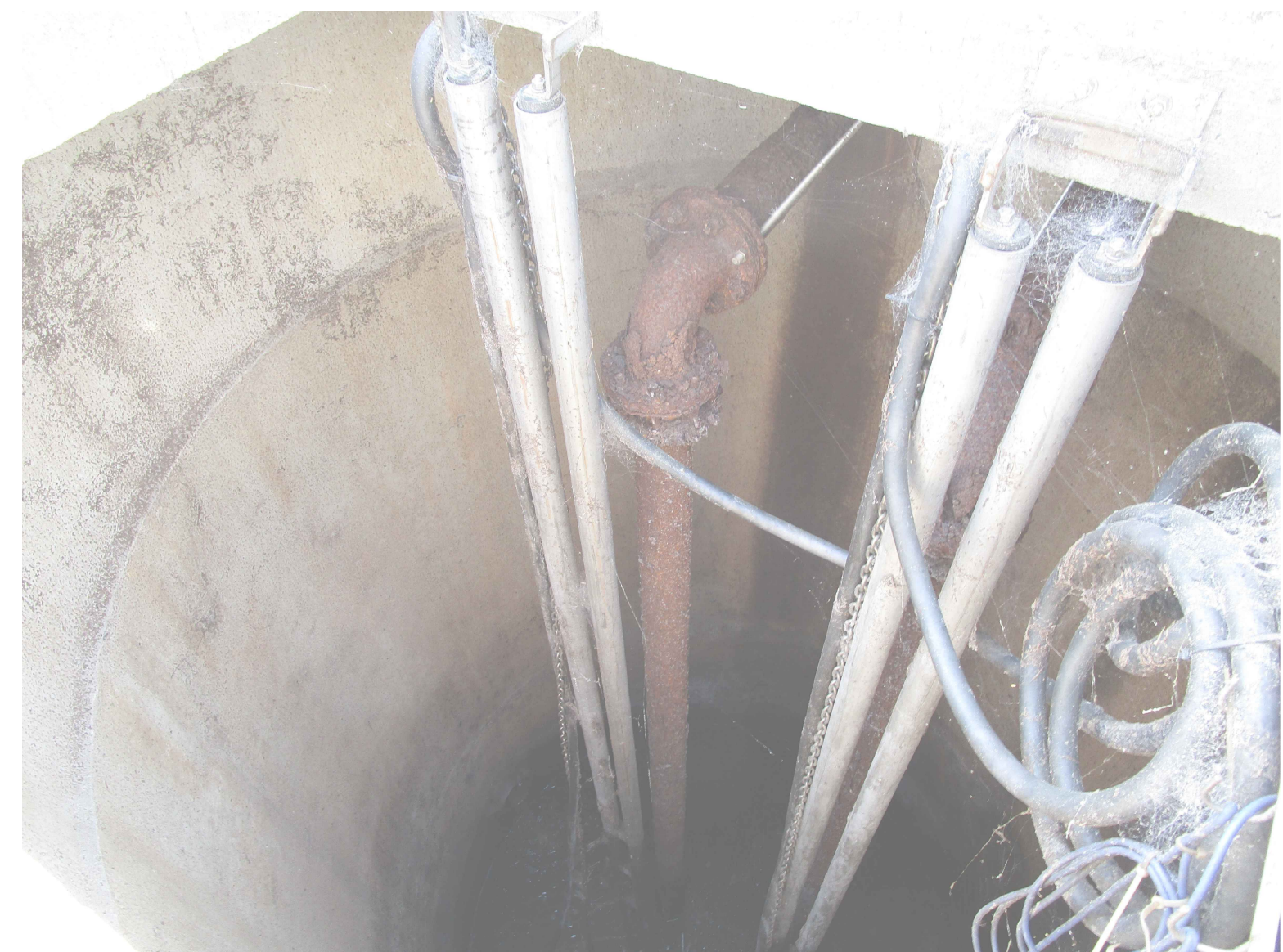
PHOTO-2 LOOKING DOWN INTO WET WELL
