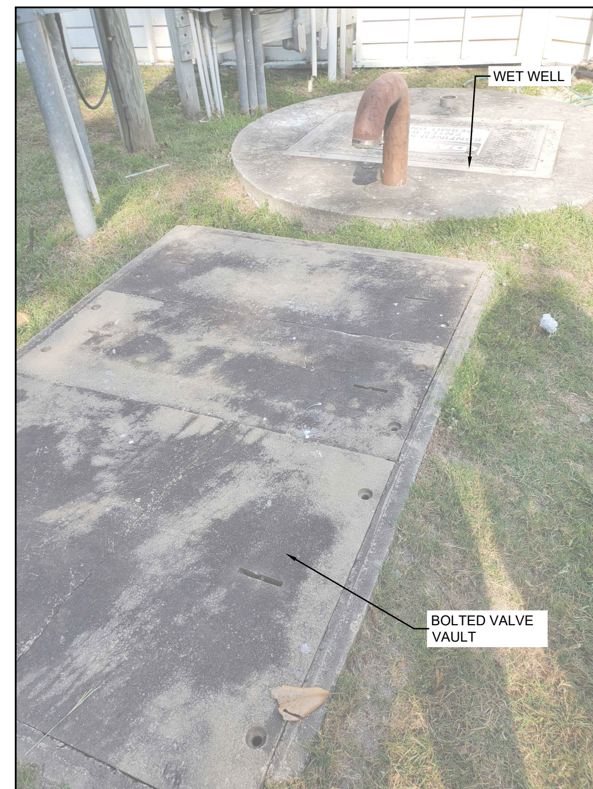
PHOTO-4 LOOKING EAST ACROSS VALVE VAULT AND WET WELL
