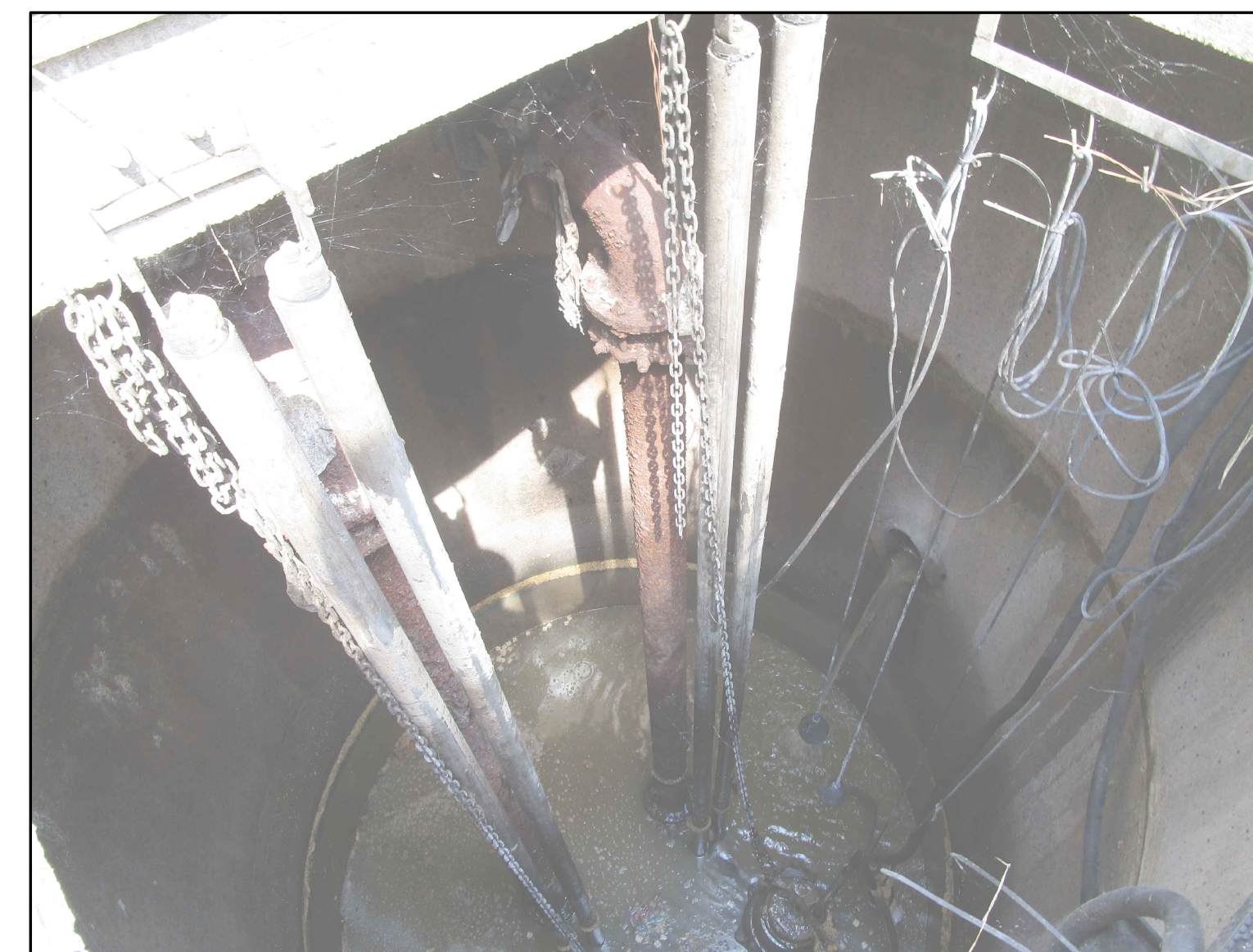
PHOTO-2 LOOKING INTO WET WELL
