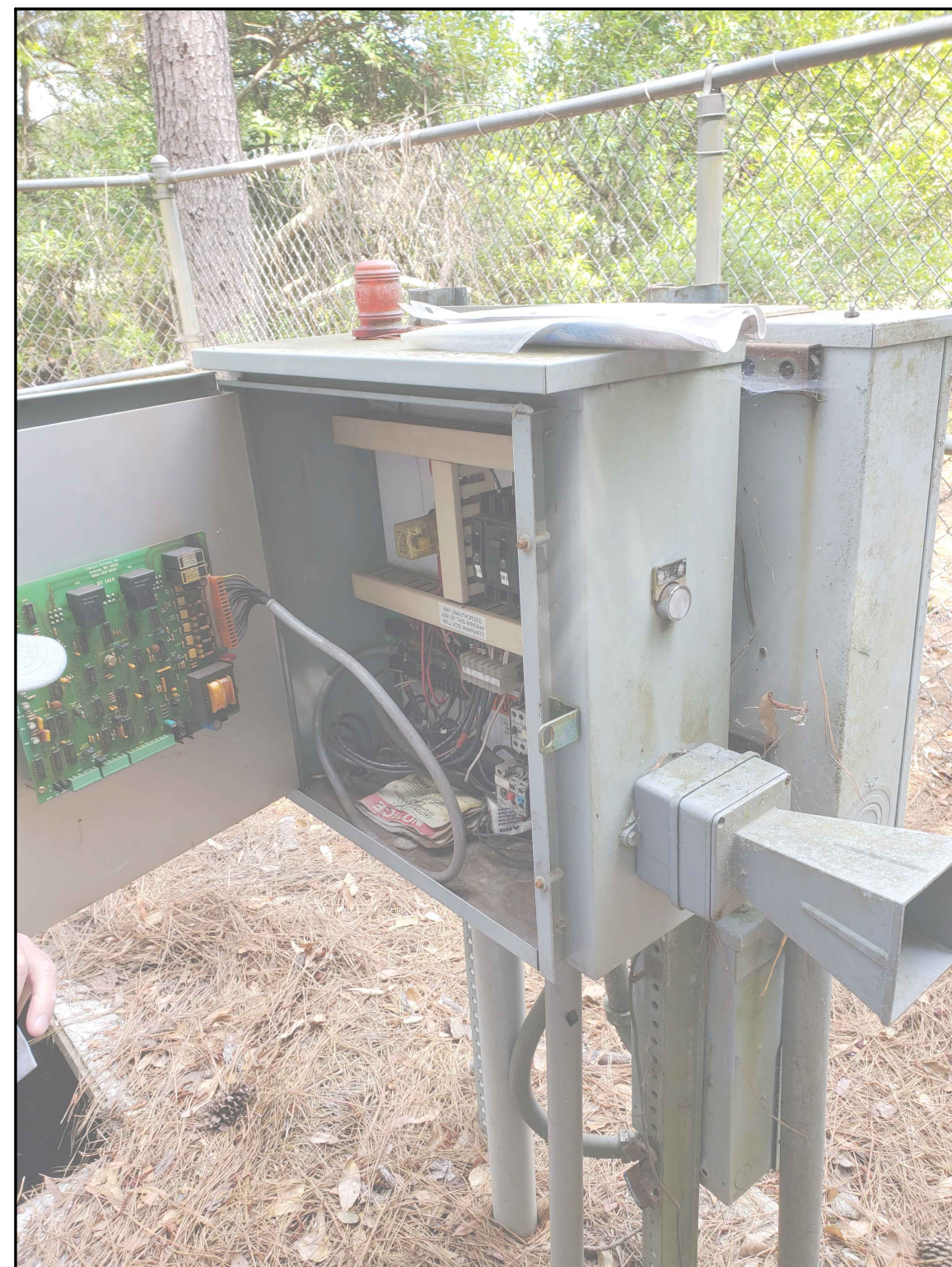
PHOTO-8 LOOKING NORTHWEST AT CONTROL PANEL
