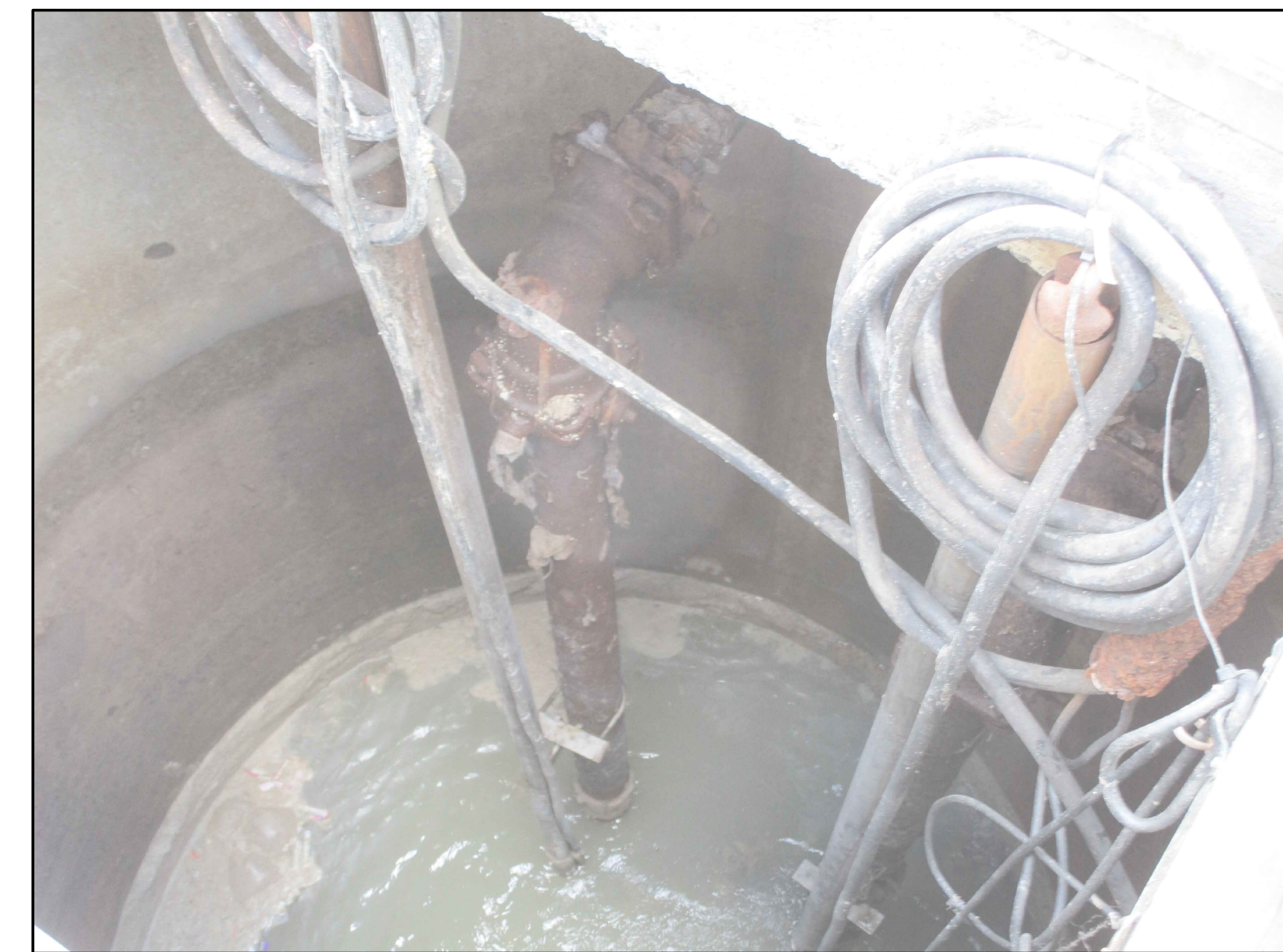
PHOTO-2 LOOKING INTO WET WELL
