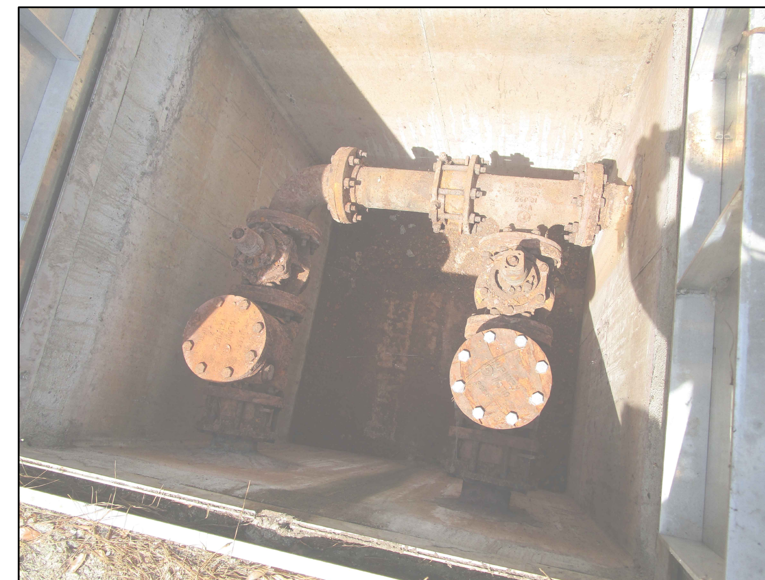
PHOTO-3 LOOKING INTO VALVE VAULT
