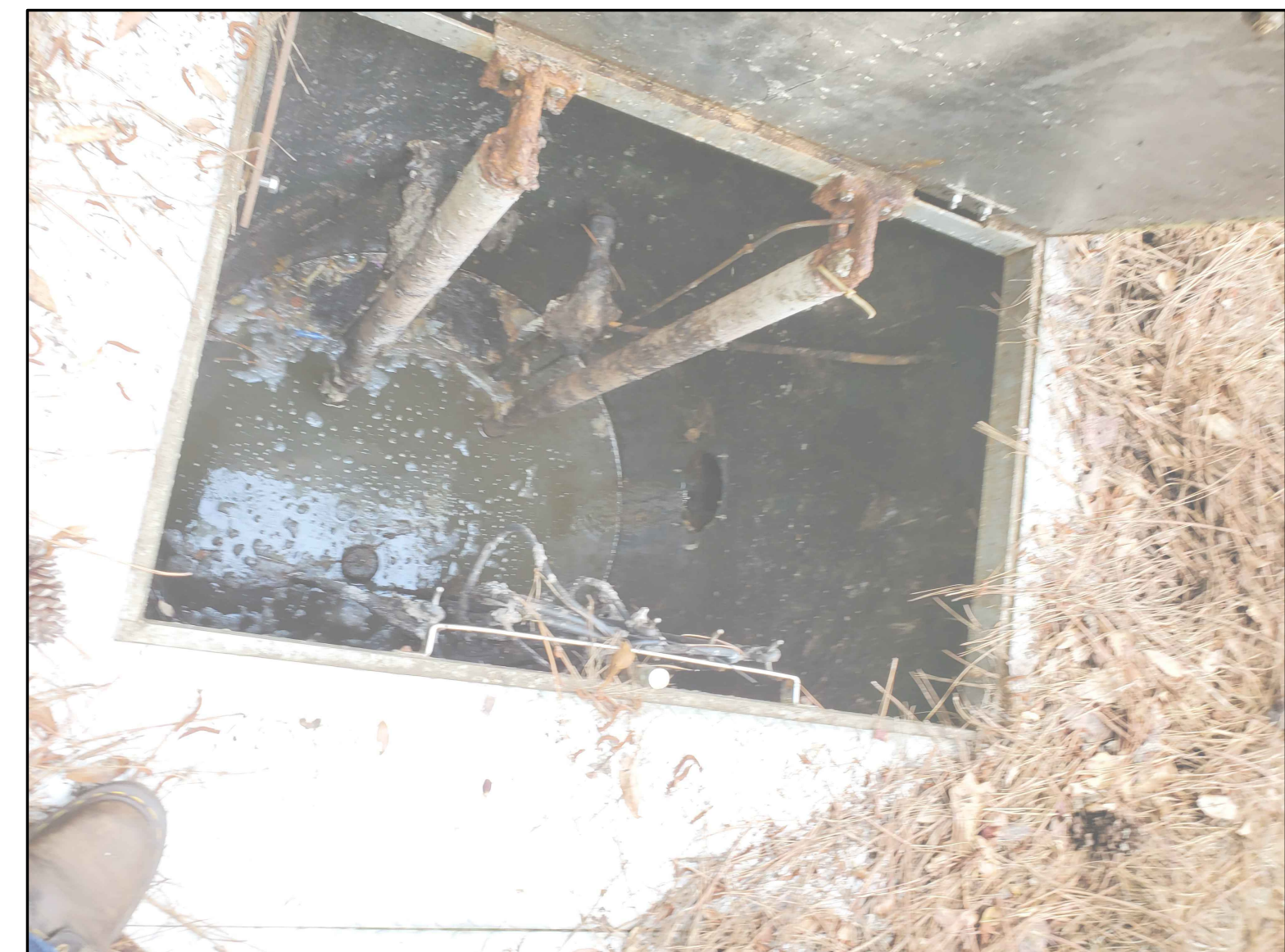
PHOTO-9 LOOKING WEST AT WET WELL
