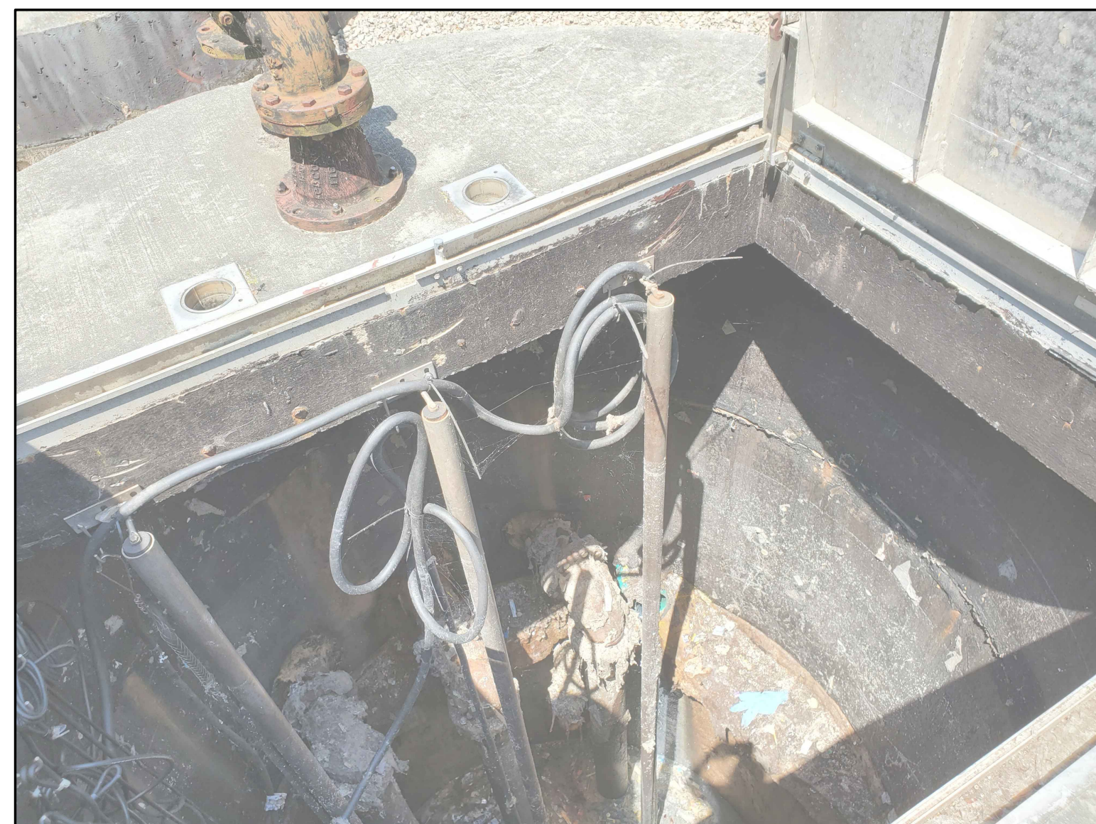
PHOTO-7 LOOKING DOWN IN WET WELL
