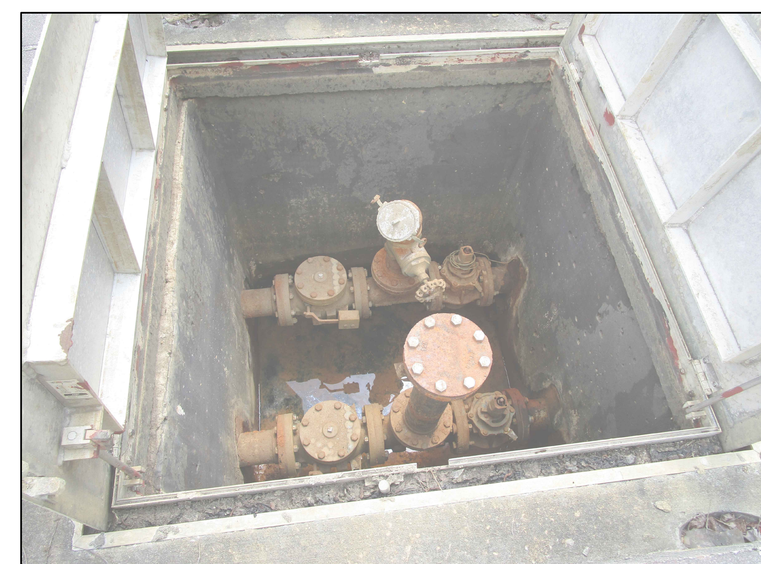
PHOTO-3 LOOKING INTO VALVE VAULT
