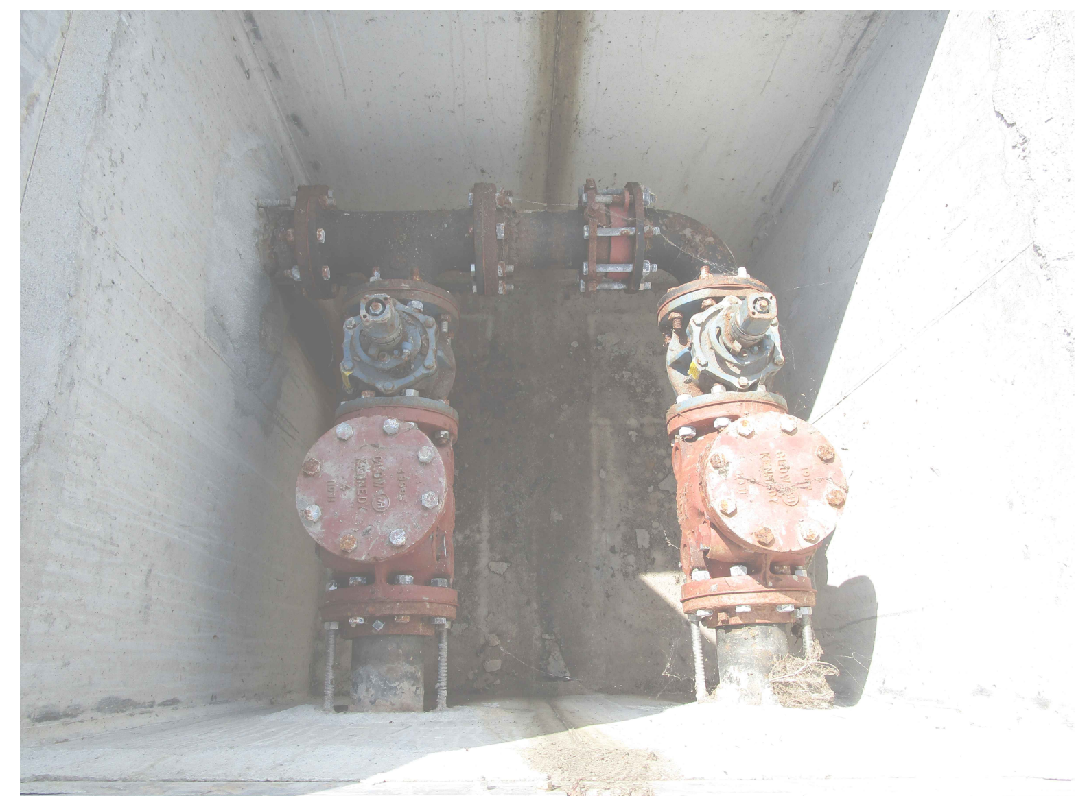
PHOTO-3 LOOKING DOWN INTO VALVE VAULT
