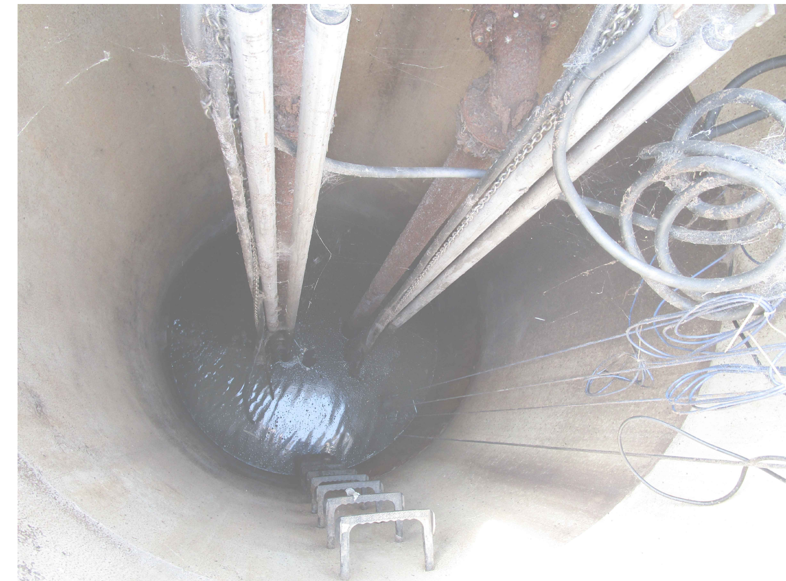
PHOTO-1 LOOKING DOWN INTO WET WELL
