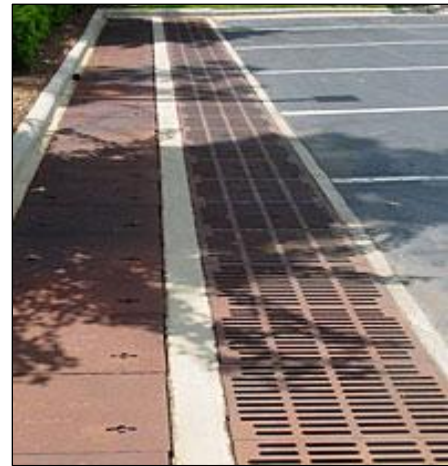
Figure 5-3 Perimeter Sand Filter in Parking Lot Source: Clean Water Education Partnership
