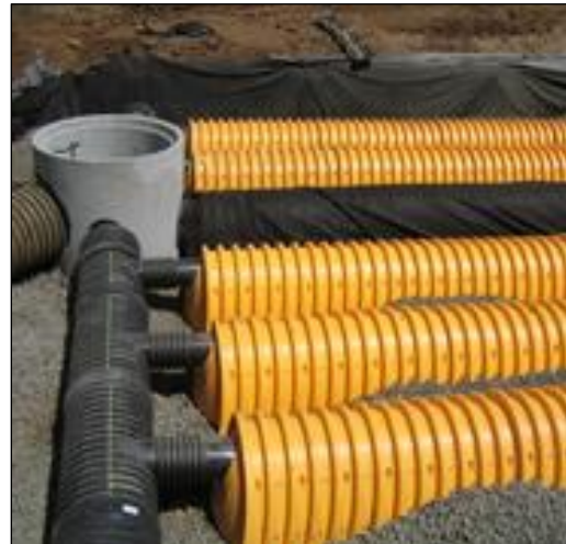
Figure 5-4 Underground Detention System Source: Stormtech
