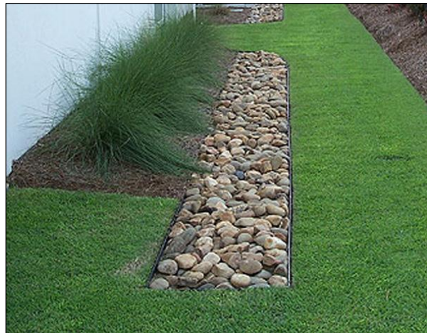
Figure 5-4 Infiltration Trench Source: Bellingham, WA
