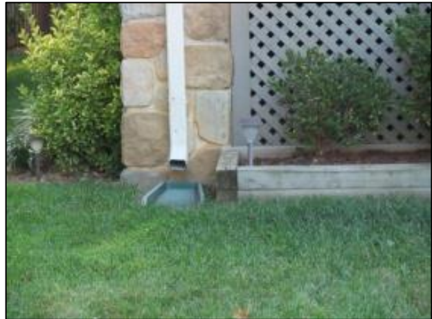
Figure 4-5 Simple Downspout Disconnection
